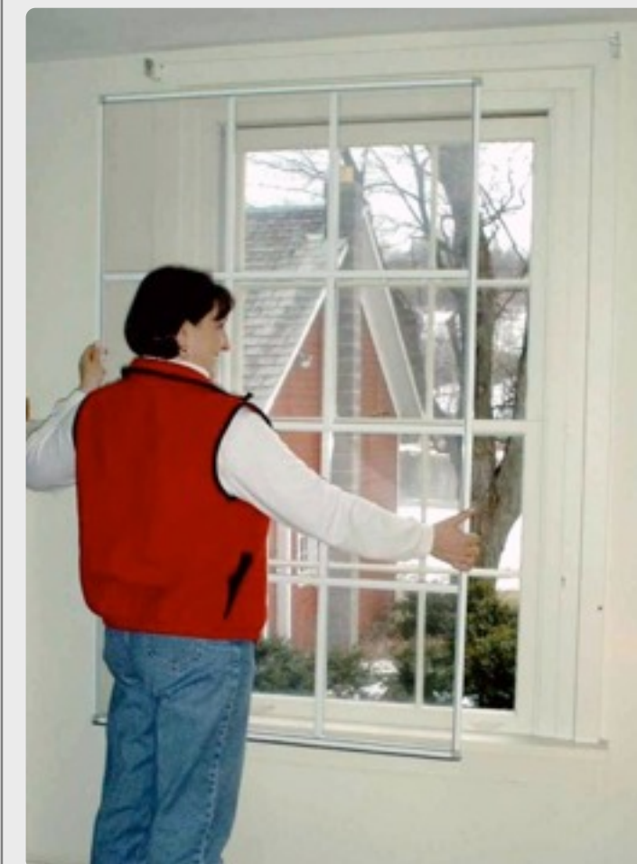
An Advanced Energy Panel being installed
