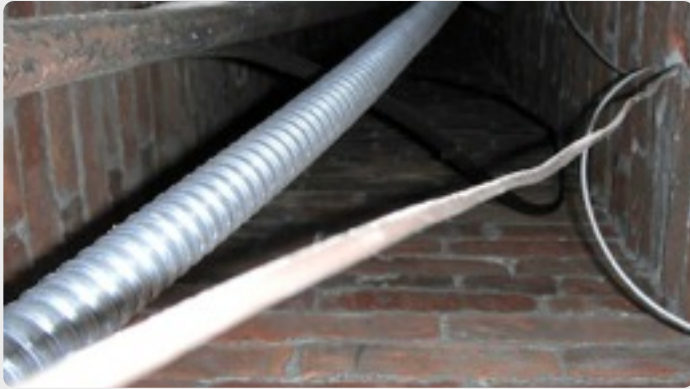
Large wire chase shown from the attic looking down into the recesses of the building. Standing above it, it was easy to feel the heat gushing out of the building.
