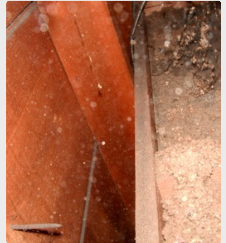
The gap in the framing for a gable end is sometimes quite obvious.
