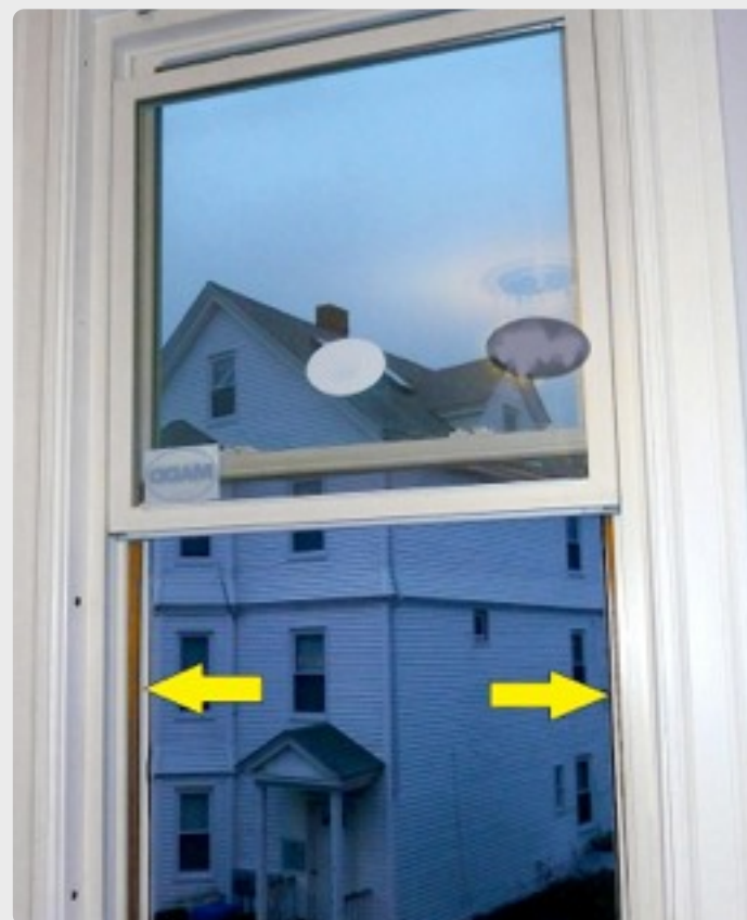
Sash props prop the upper sash up into position so it doesn't sag.
