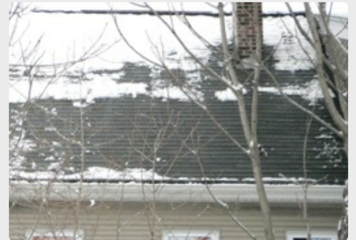
Knee wall melt on roof
