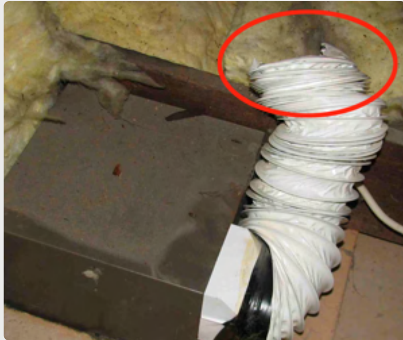
A bathroom fan where the vent isn't connected to the outside can dump a lot of water into your attic.
