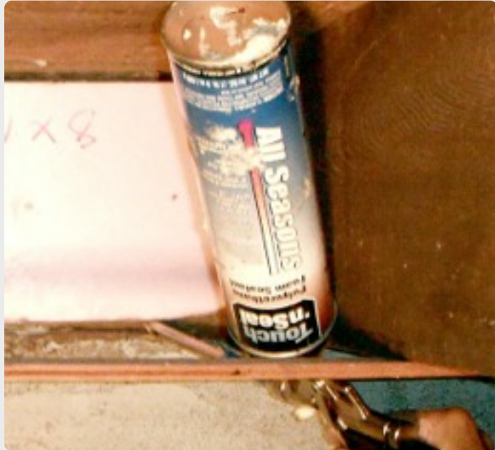
The correct way to hold the spray foam gun is with the can on top.
