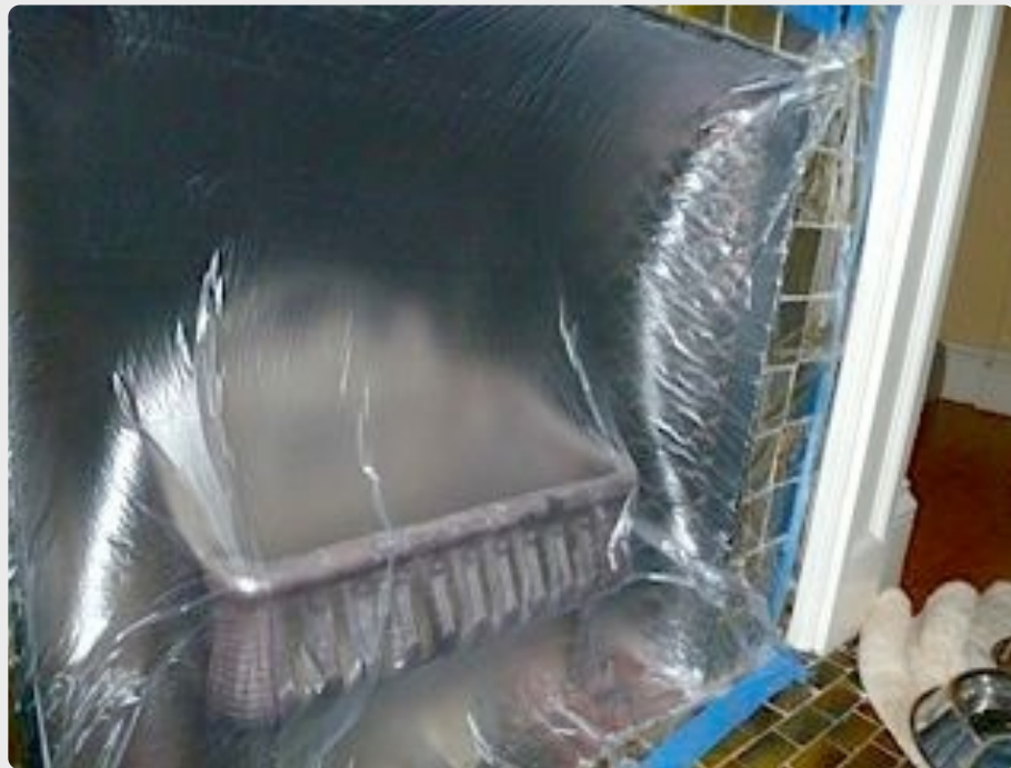
Tape a sheet of plastic over a fireplace with the damper open in order to see how much an open damper literally sucks.
