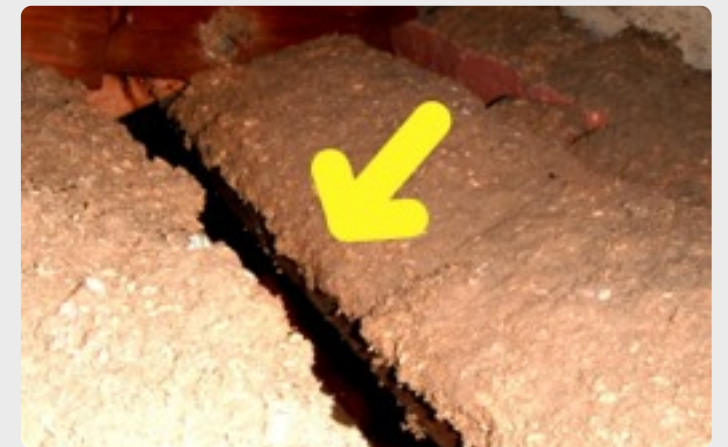
Open wet wall as seen from the attic
