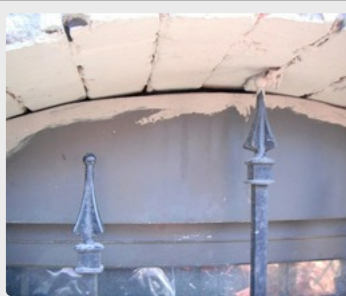
See the large crack between the bricks and the curved metal at the top of the window? It should be caulked.
