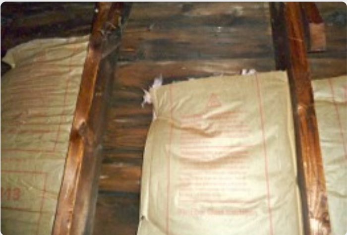
Fiberglass batts should fit neatly in between the joists to fill up the space entirely. This is a very bad insulation job.
